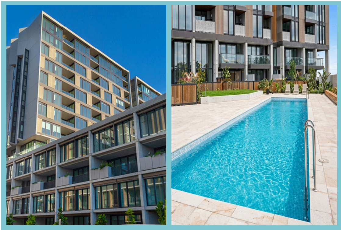
Multi Scheme Residential Towers - Ryde Gardens, North Ryde 1-5 Network Place, North Ryde NSW 2113
